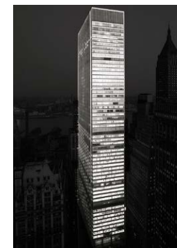
Skidmore, Orwings & Merrill (SOM) 28 Liberty Downtown 1963 57 FL 2,215,030 SF NA
